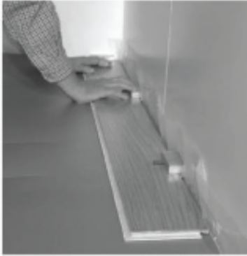
4. Start in corner positioning first board with 1/2” expansion spacers.
