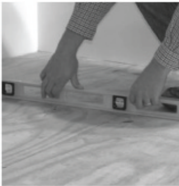
2. Make sure the floor is level and dry.
