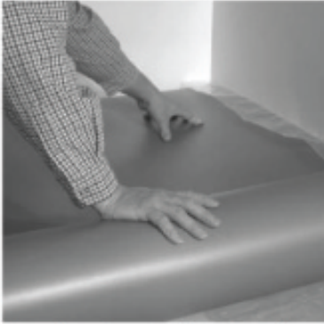
3. Roll out the underlayment, a few rows at a time to prevent tearing.
