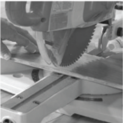
9. The cut board from the first row is used to start the second row.
